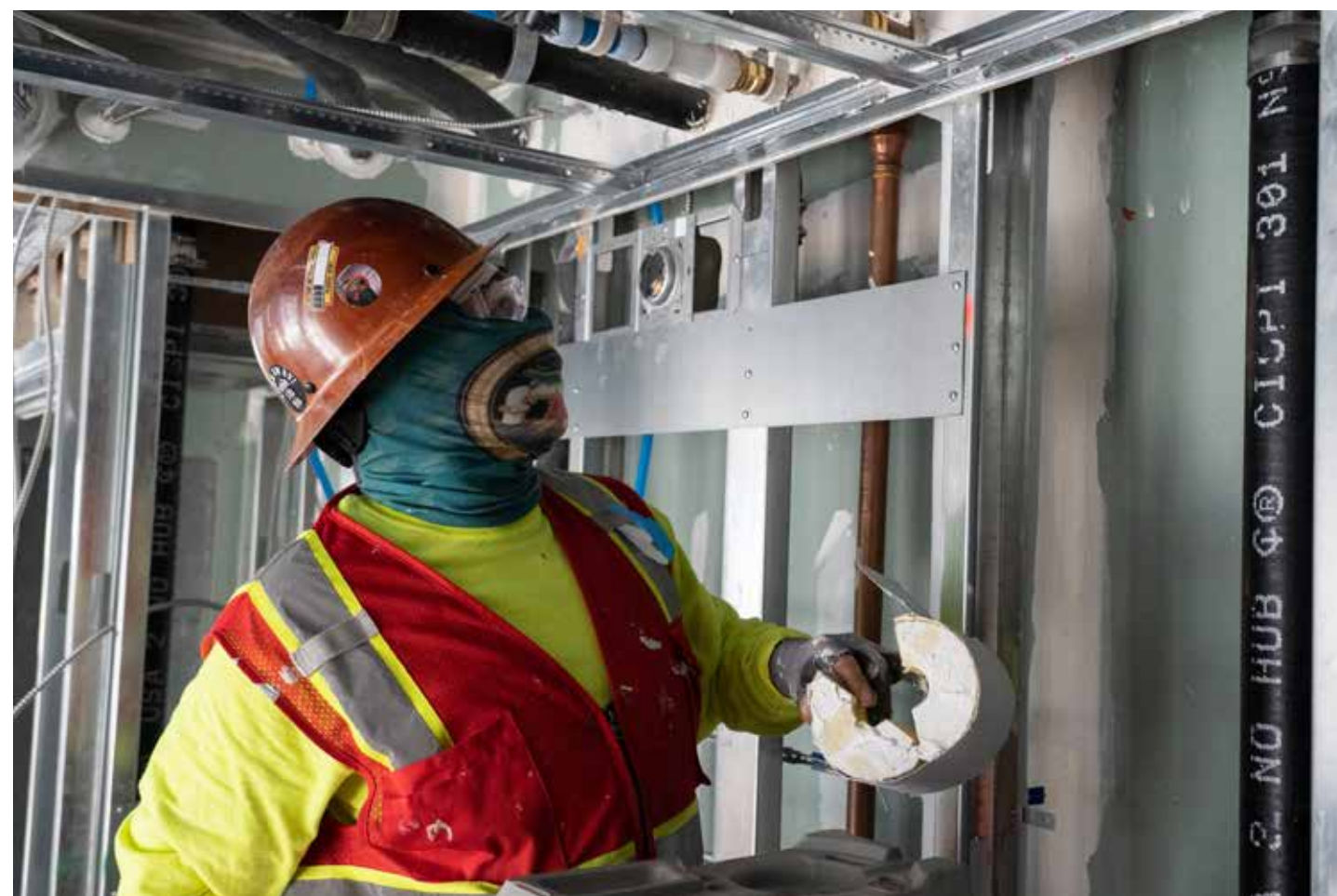
Many Building Trades locals are already working with "green" techniques that save energy. Here, Francisco Guzman of Heat & Frost Insulators Local 5 insulates hot water pipes at The Grand in Downtown LA.
