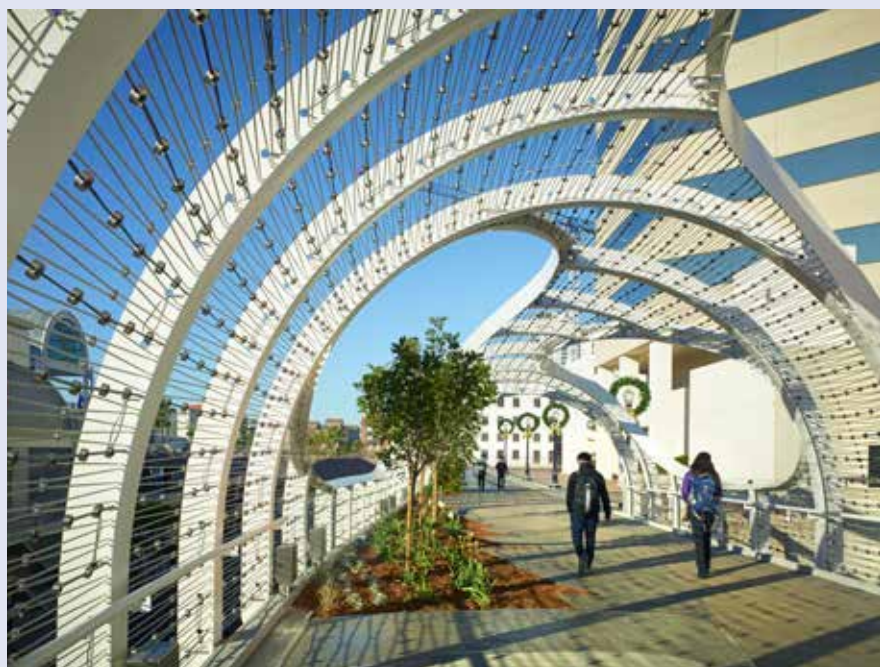
The bridge was constructed with a top frame of 76 custom-welded bent-steel ribs.
