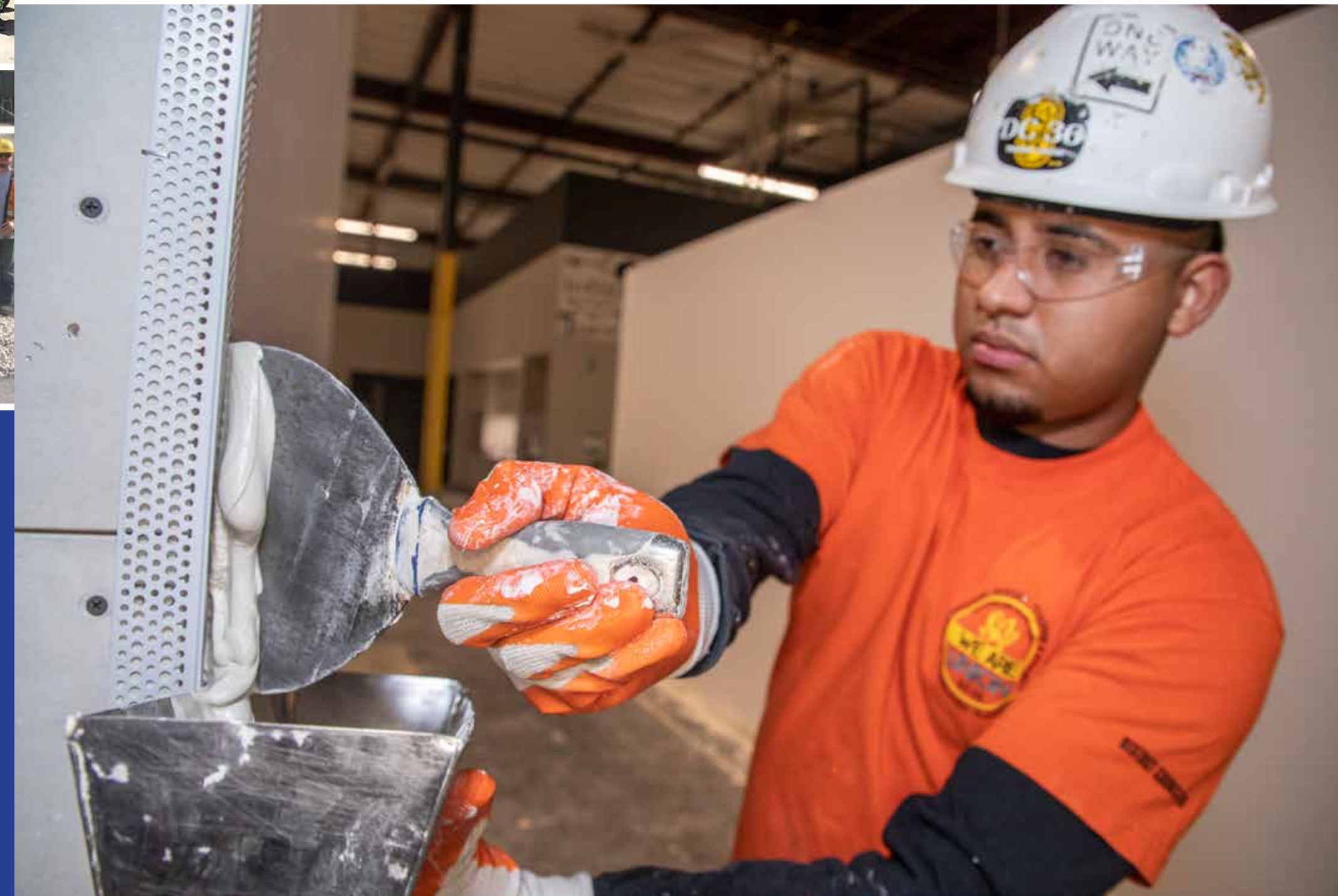
Local 1136 apprentice Erick A. Lopez shows what he's learning as he carefully applies joint compound, known as "mud."
