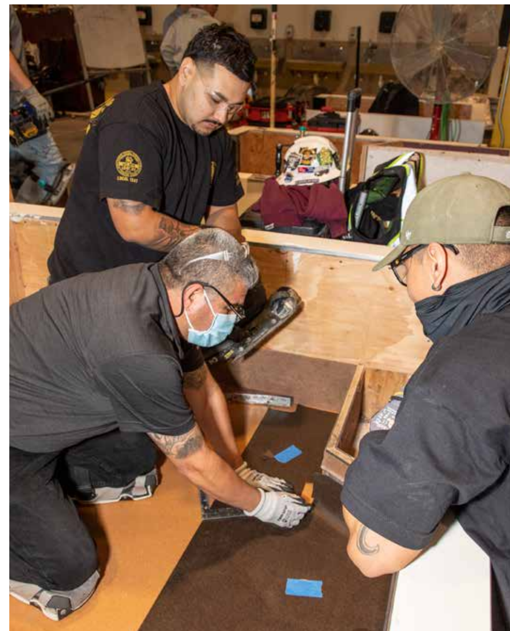
Floor Covering apprentices learn pattern scribing on a cove flooring installation.
