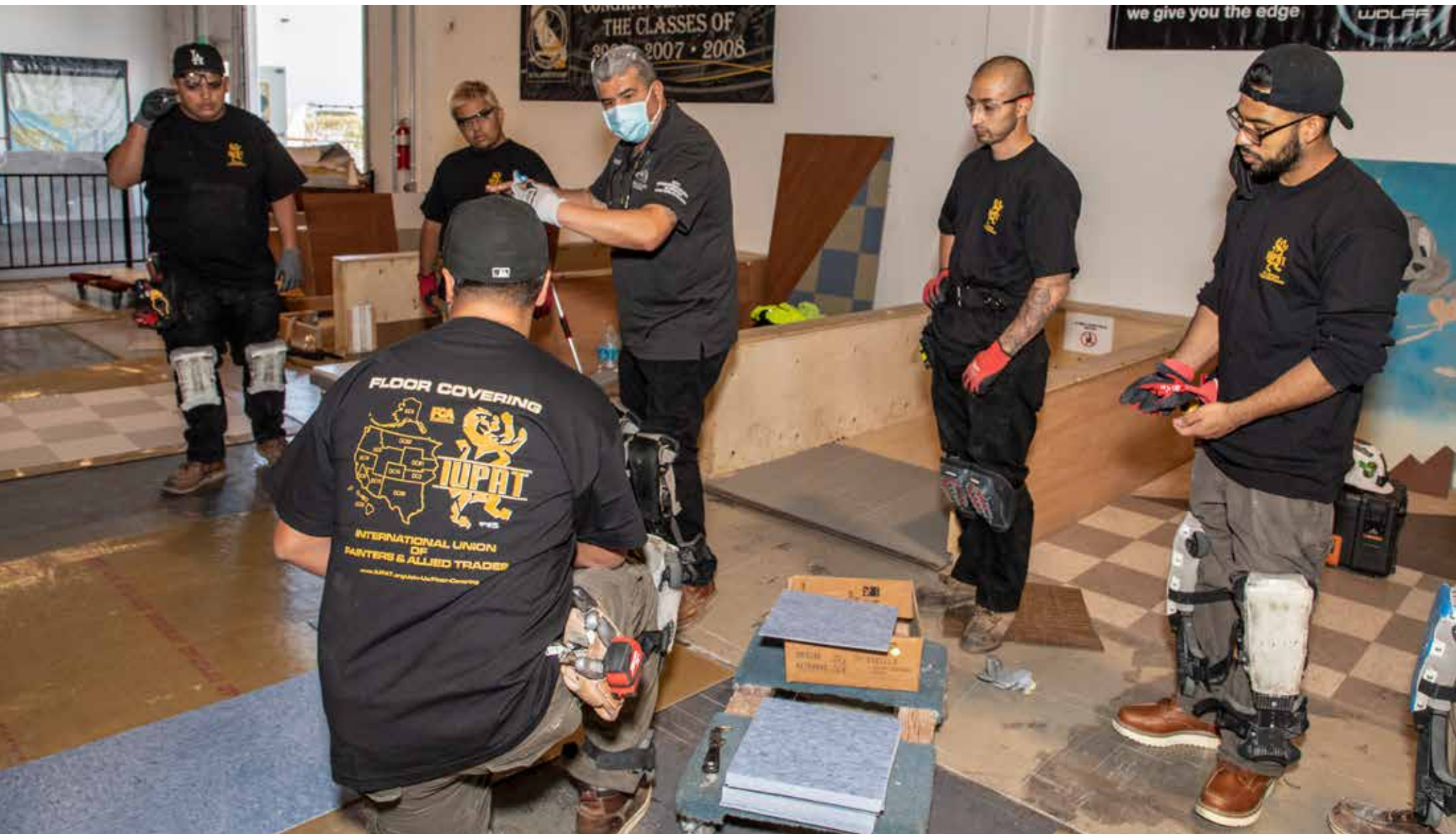
Instructor Luis Viramontes explains the proper layout of VCT (vinyl composite tile) flooring.
