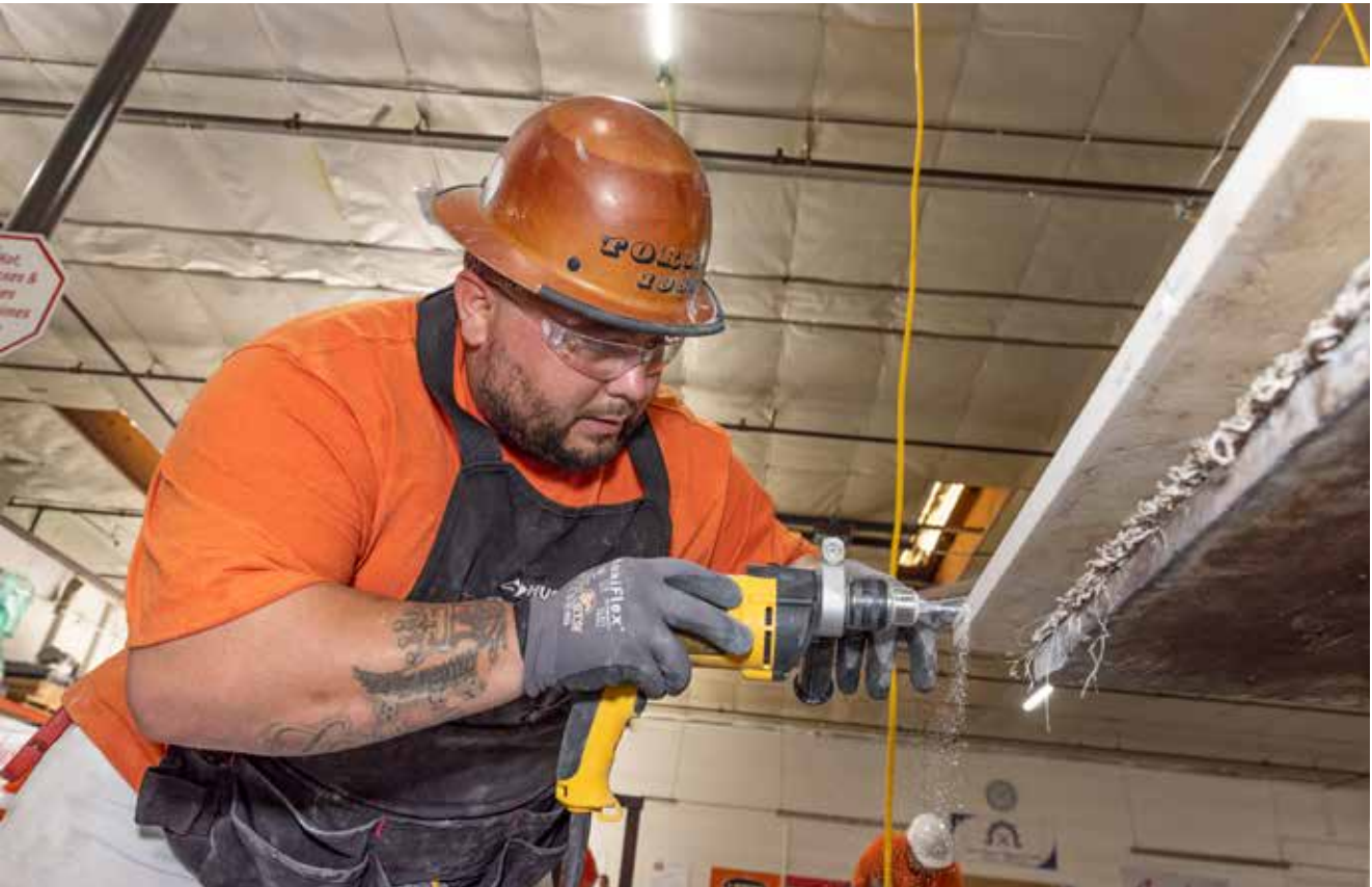
BAC Local 4 Marble Mason apprentice Joseph Torres drills holes for a “spot and anchor” installation of a marble panel.
