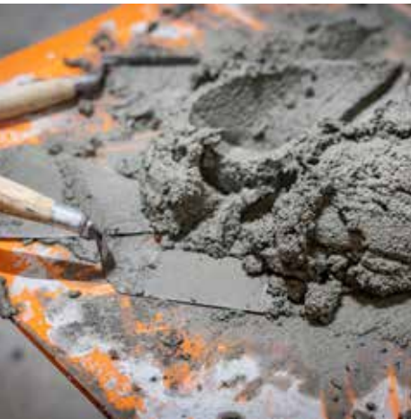
Brick mortar is mixed and ready.
