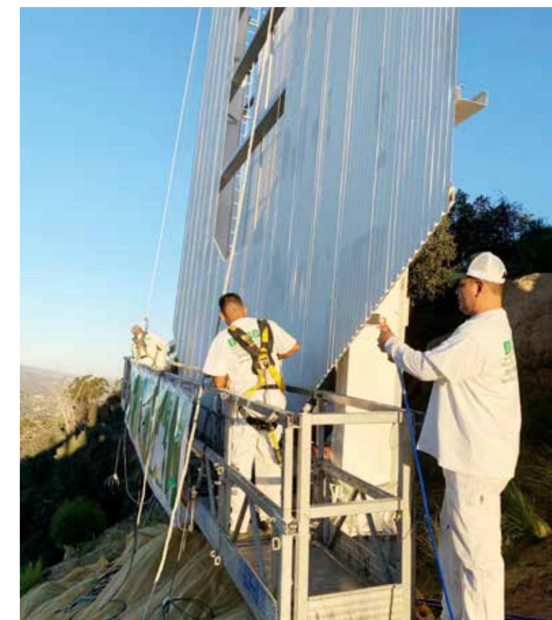
The letters are washed and primed before painting.
