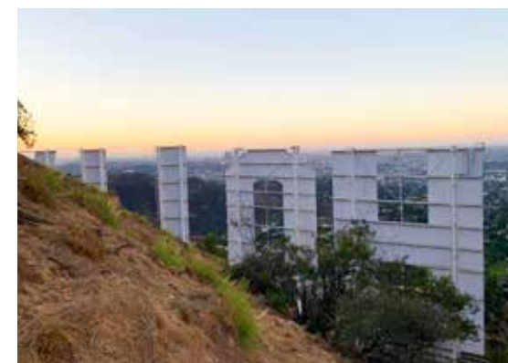
The sign is made of corrugated steel.
