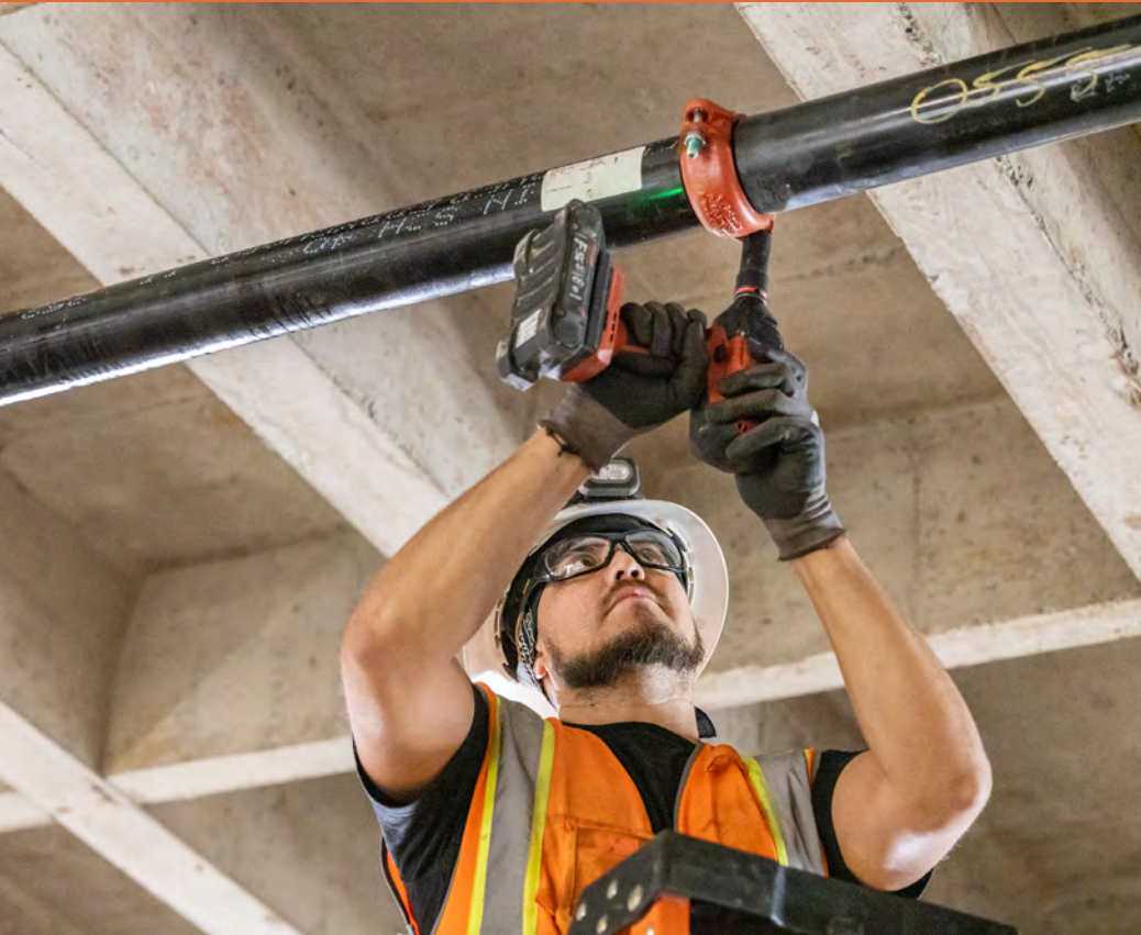
Calvin Guerrero, UA Local 709 Sprinkler Fitters apprentice, installs a main for sprinkler heads.
