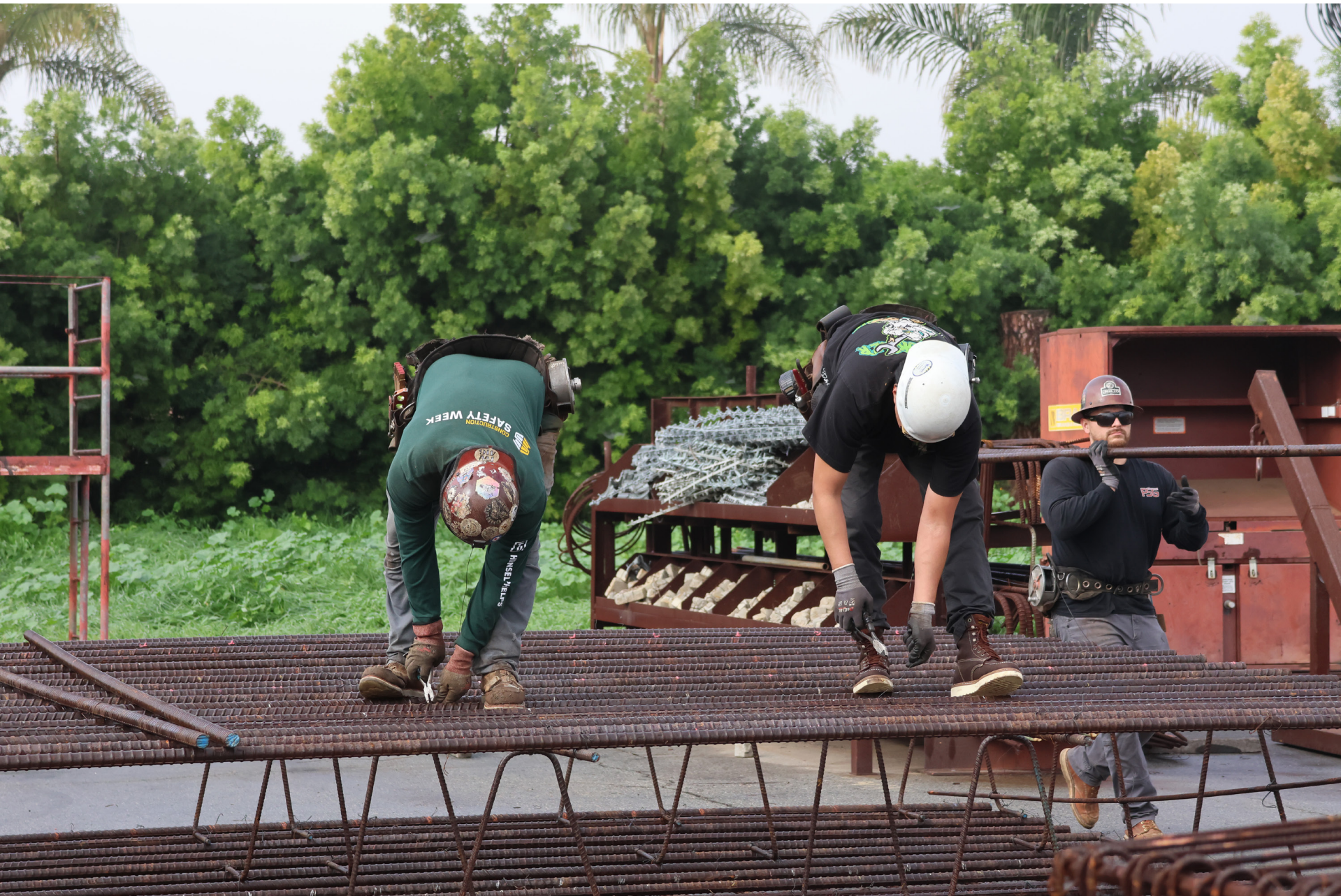
Apprentices carrying rebar and securing a rebar structure with ties.
