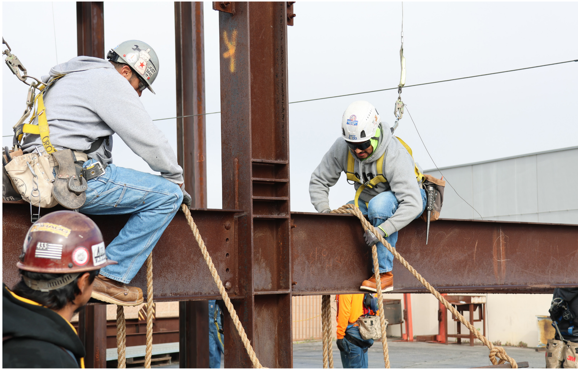
Left and right, Apprentices adjusting rope as they lift iron beams on the training structure.
