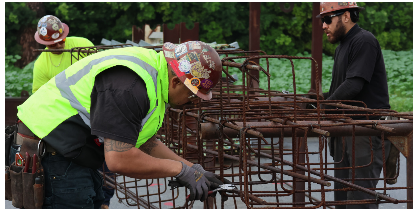
Apprentices securing a rebar structure with ties.
