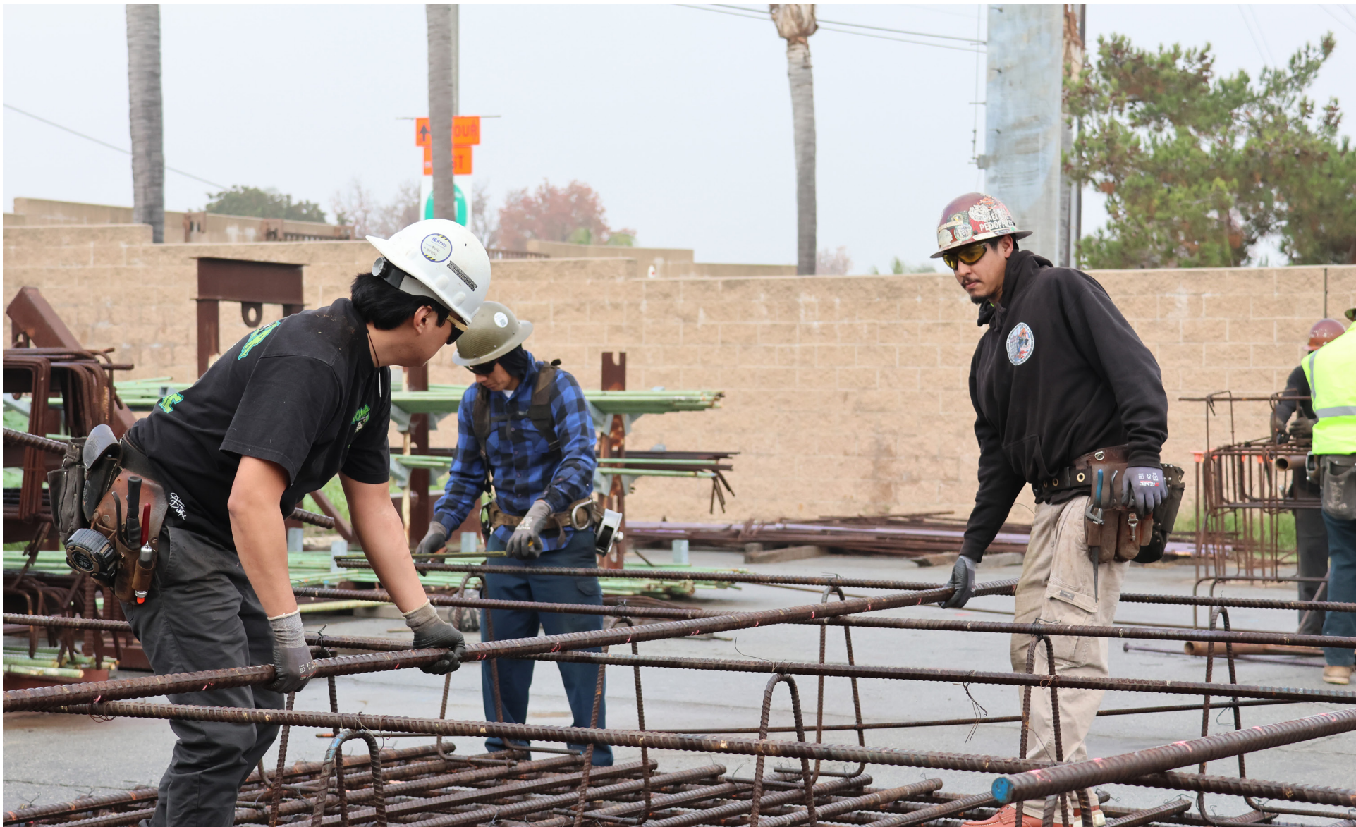
Apprentices assembling a rebar training structure.
