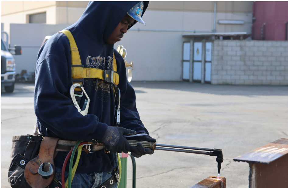
Apprentices using blowtorch on iron beam.
