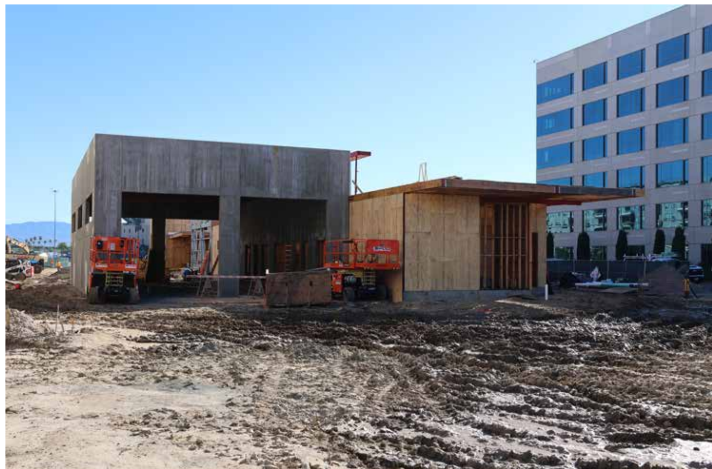
Full view of the fire station under construction.
