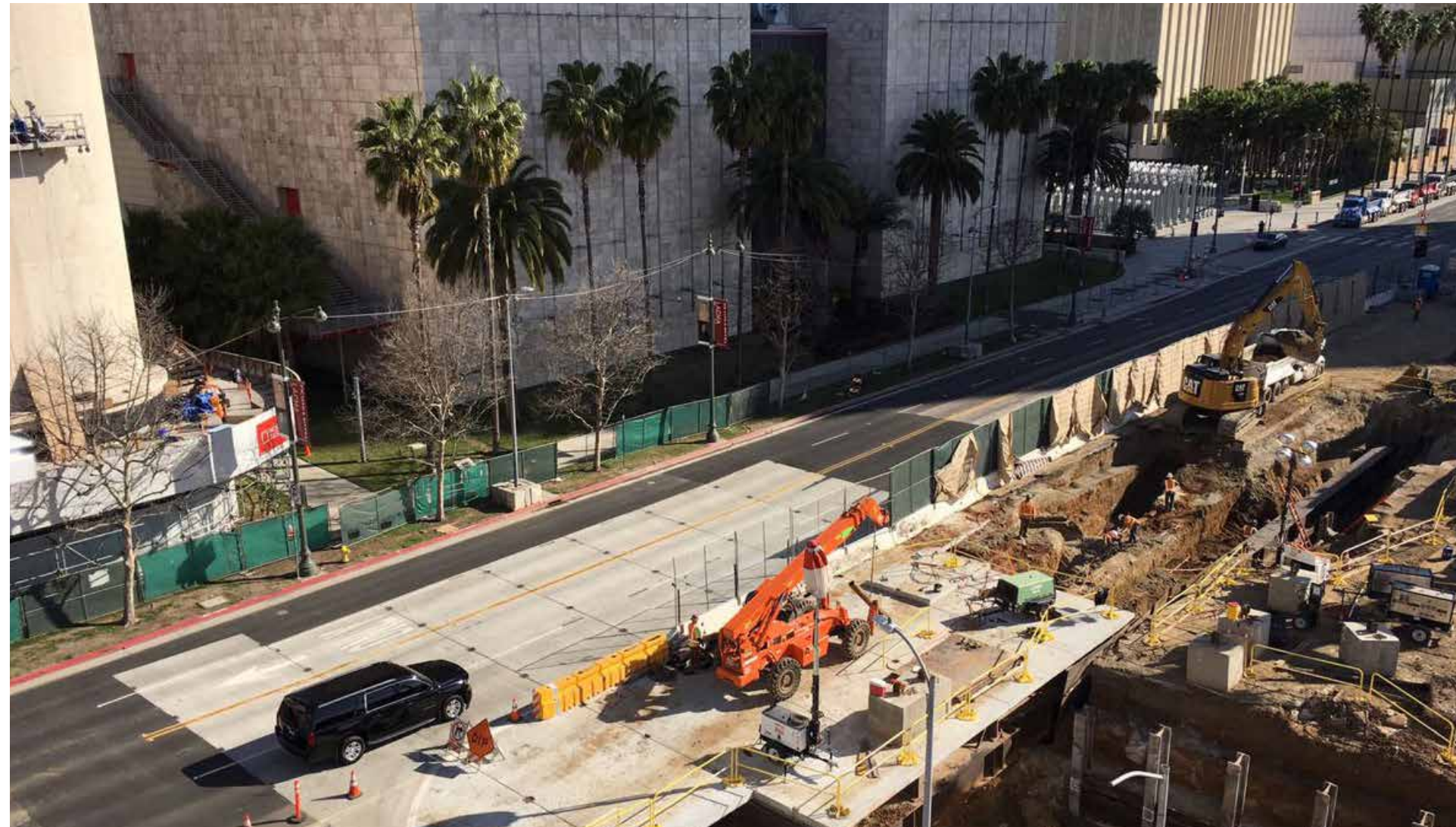
Metro D Line construction near LACMA.
