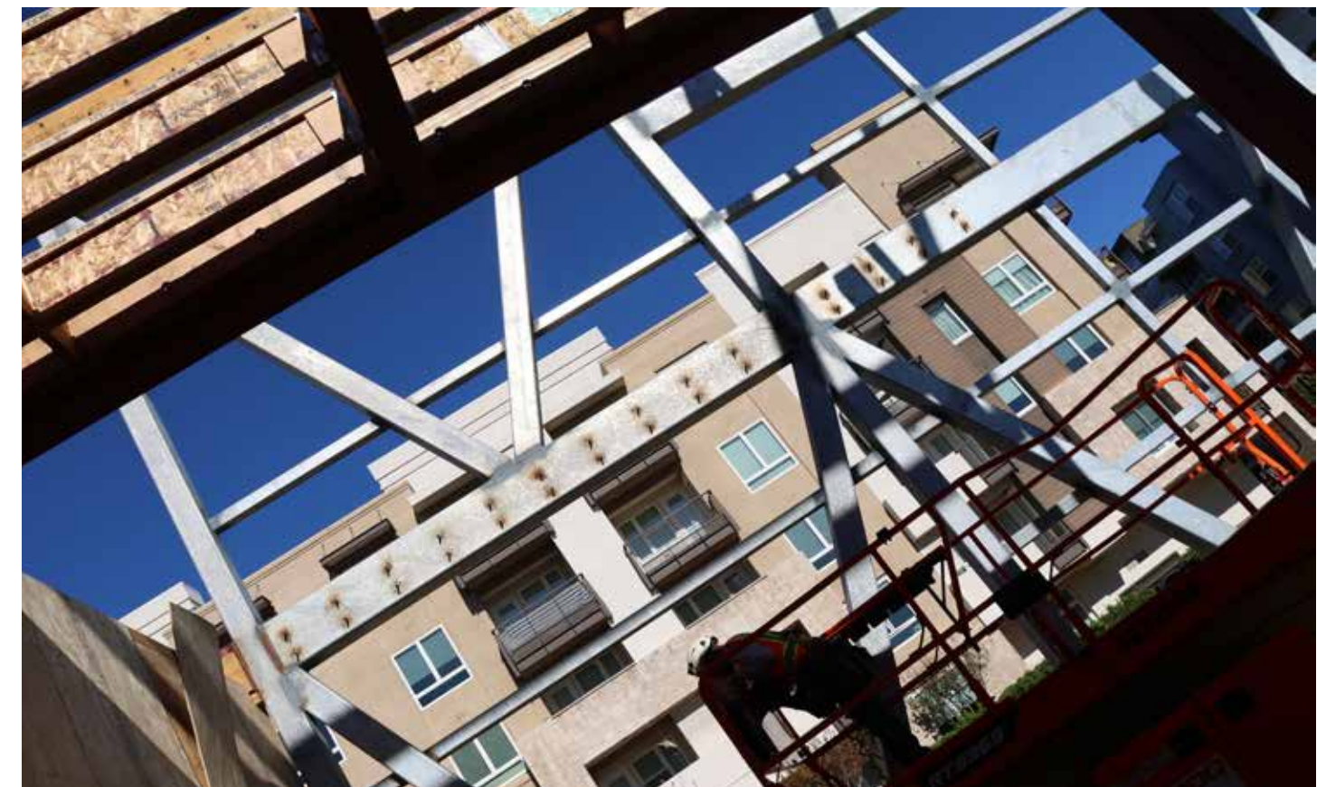
View from the inside of the fire station.
