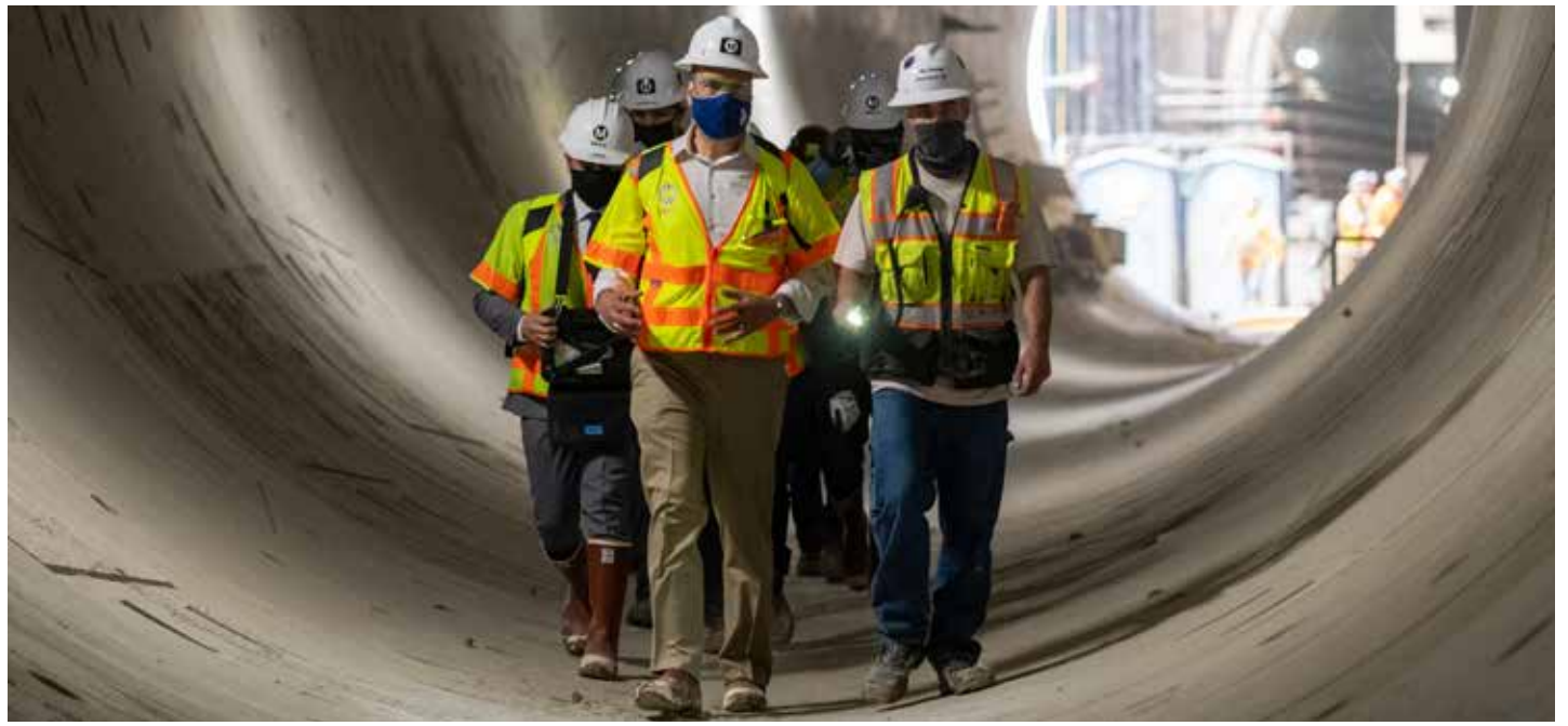
Construction workers walking through a train tunnel.
