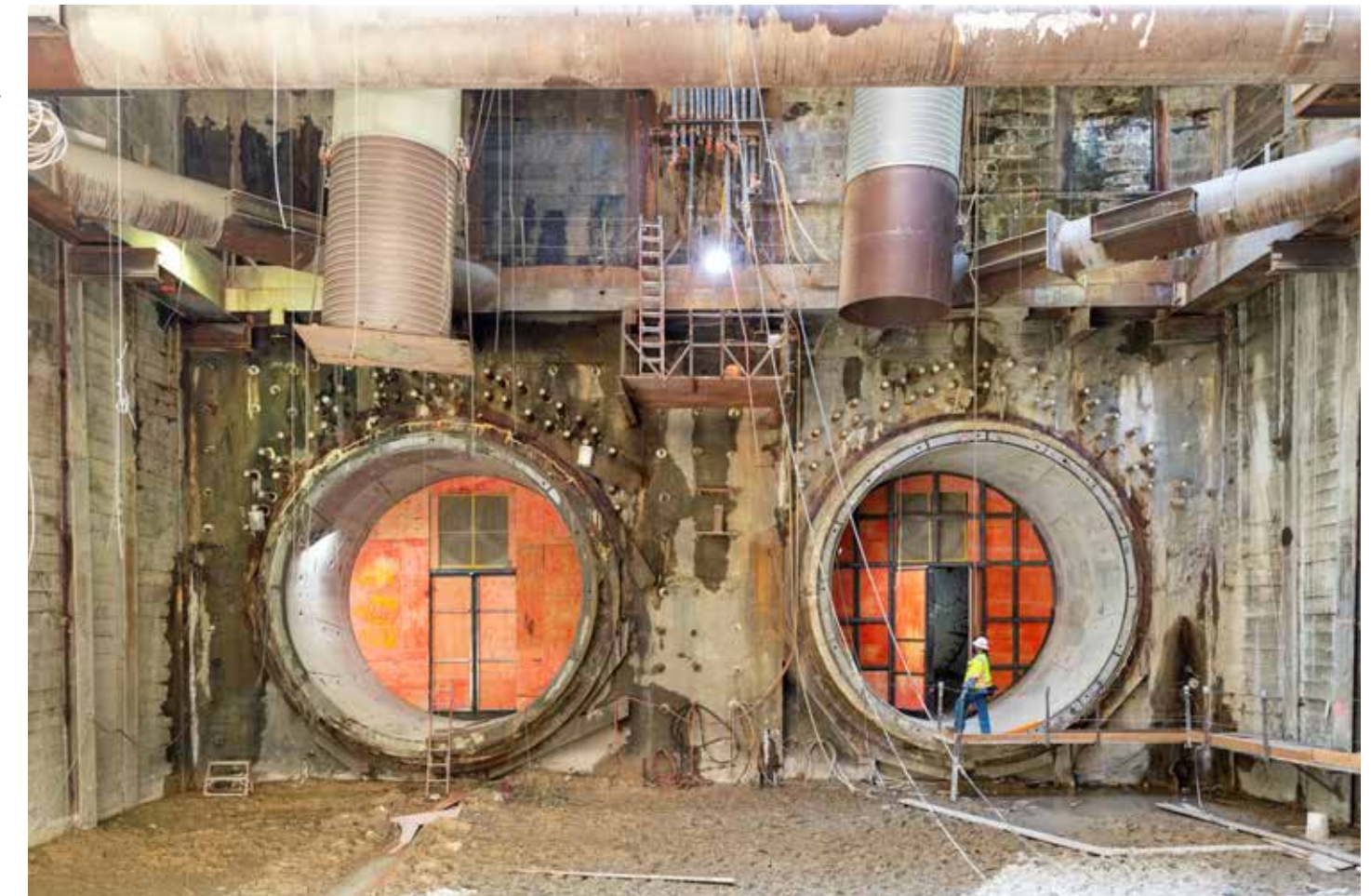
Construction workers walking through a train tunnel.
