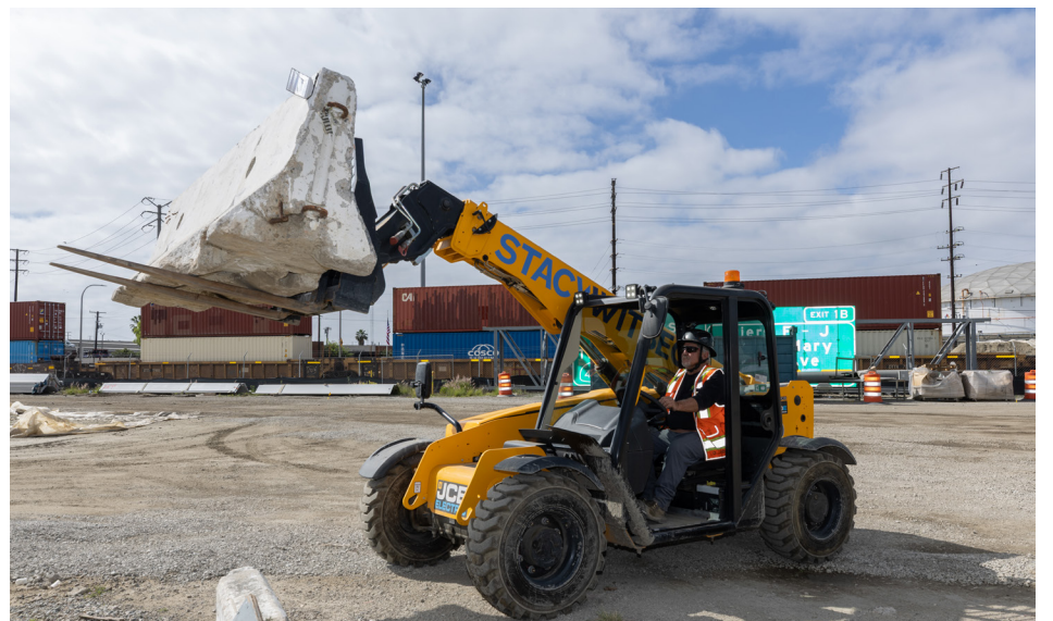
Crews use zero-emission equipment as part of infrastructure work at the Port of Long Beach. Courtesy of the Port of Long Beach.
