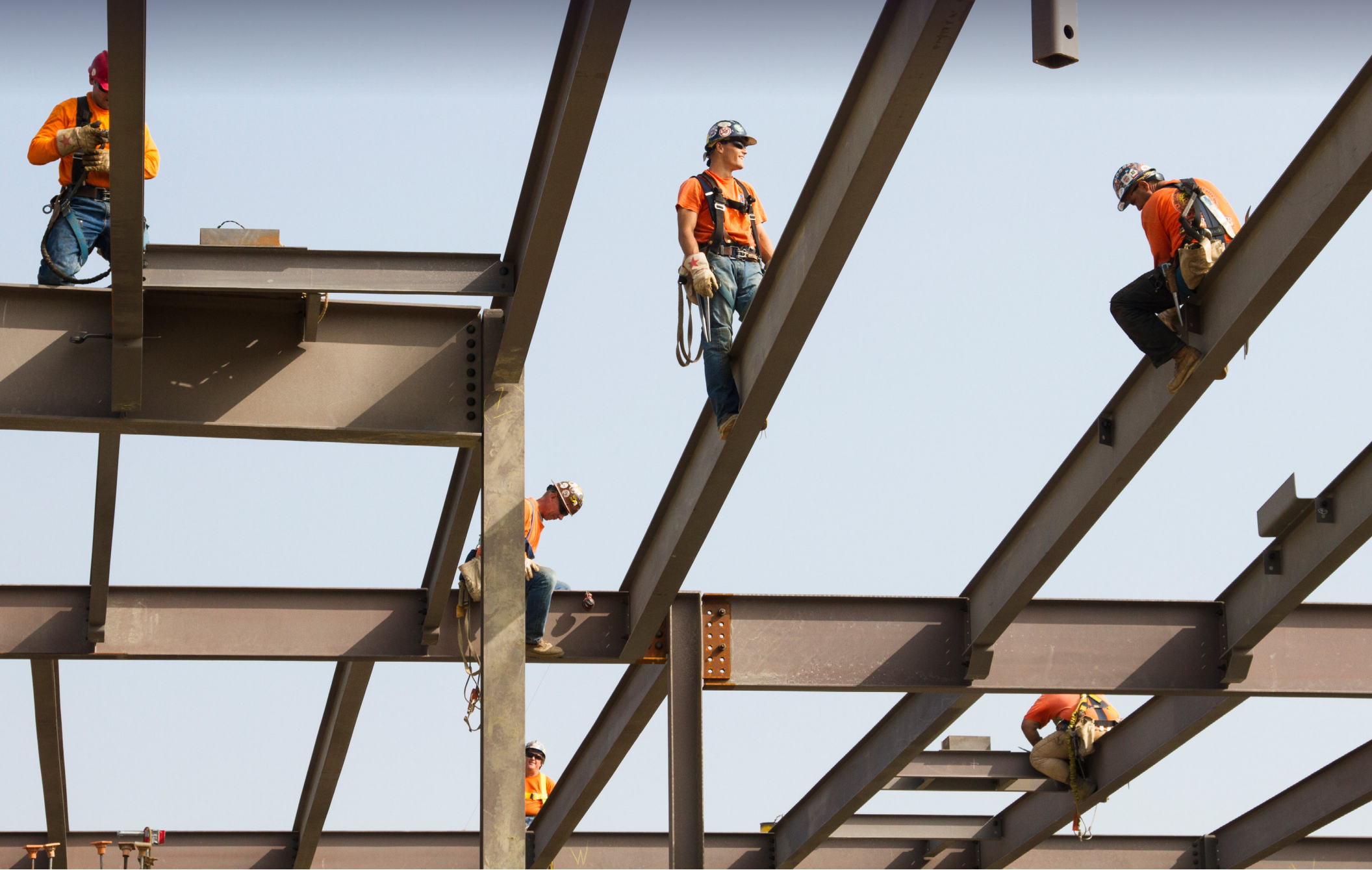
Structural ironworkers install steel framing at the Port of Long Beach. Courtesy of the Port of Long Beach.
