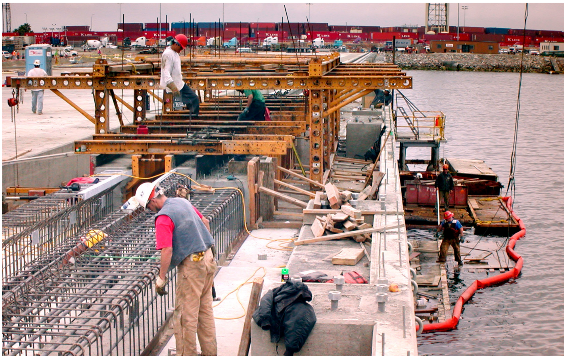
Skilled trades workers build the marine infrastructure that supports Port of Long Beach operations. Courtesy of the Port of Long Beach.
