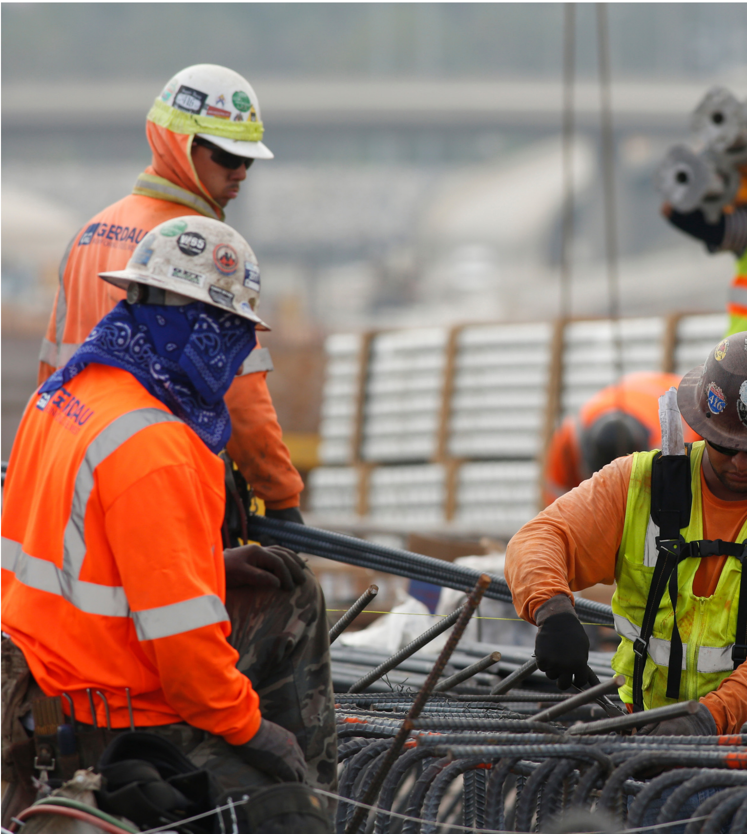
Reinforcing ironworkers working at the Port of Long Beach. Courtesy of the Port of Long Beach.
