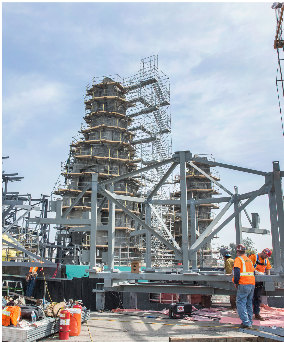
Members of Pipe Trades UA Local 582 working at Disneyland.
